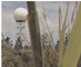
Burma reed in foreground with Doppler radar in background
